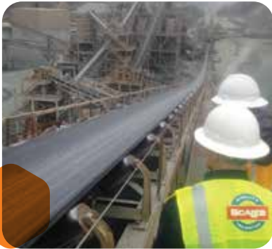
Conveyer Belt Installation
