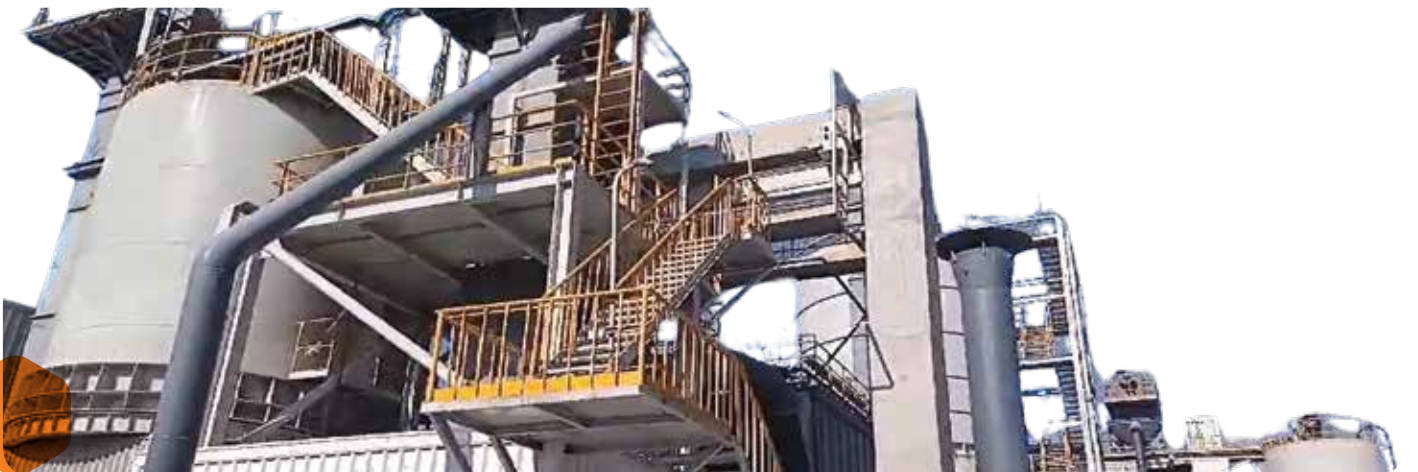
Faisal Engineering Services marks history with Pakistan's first 9000TPM White Cement Based Wall Putty Plant.
