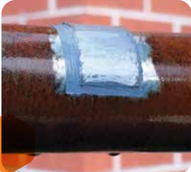
In-Situ Steel Patching
