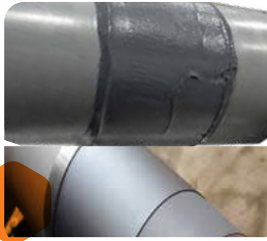
Cold Welding Shaft Rebuilding
