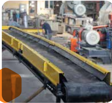
Conveyor Structure Installation
