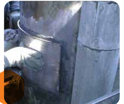
Cold Steel Bonding without heat
