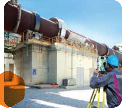
Cement Kiln Shell Inspection for Replacement
